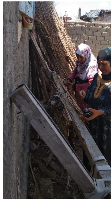
Figure 8: Couple of women working in preparing the reed fence
