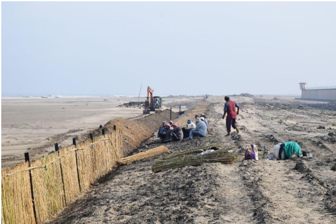
Figure 11: Land preparation activities
