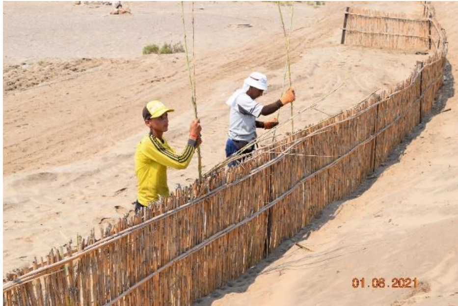
Figure 12: Activities associated with reed fences construction
